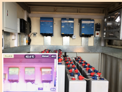
Kitonyoni mini-grid plant room 2022. Inset thermal image of inverters for performance analysis
