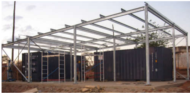
Ease of installation with multipurpose structures for PV modules, water collections and shading (Kitonyoni), Kenya.
