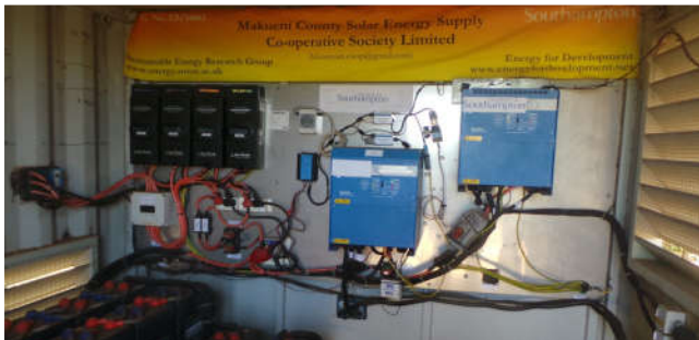
Containerised PV System. Redundancy in design with all projects with 2 inverters (master-slave) - Kitonyoni, Kenya.
